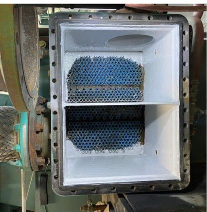
Once repaired, the unit was then coated using Belzona 1331. This coating also offers a long overcoating window that facilitated the application process for the contracting crew.
