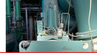
It was an easy decision for the customer to coat a larger unit as well using Belzona products. Belzona 1331 was used for this application. This is a two coat system for corrosion and erosion protection of equipment operating under continuous immersion.
